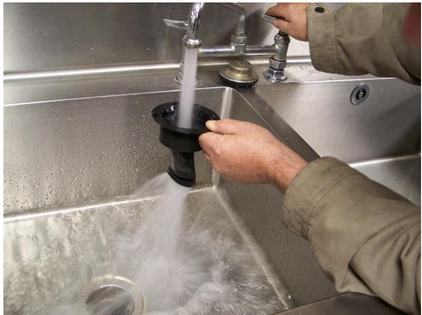
Trap guards are a simple fix for dry drains! Photo courtesy of Texas AgriLife Extension Service.
