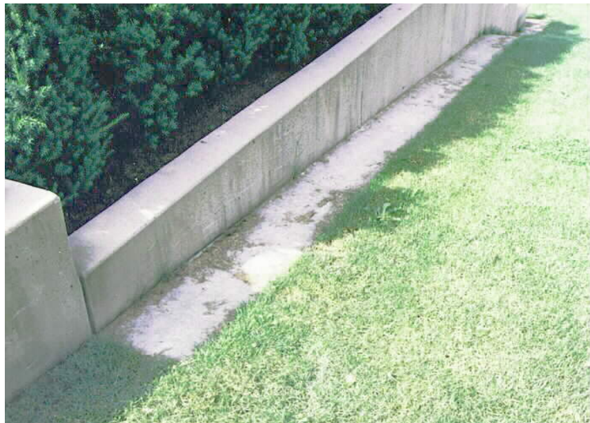
Mowing strip used to reduce pesticide use on areas that are not easily reached by mowing.
