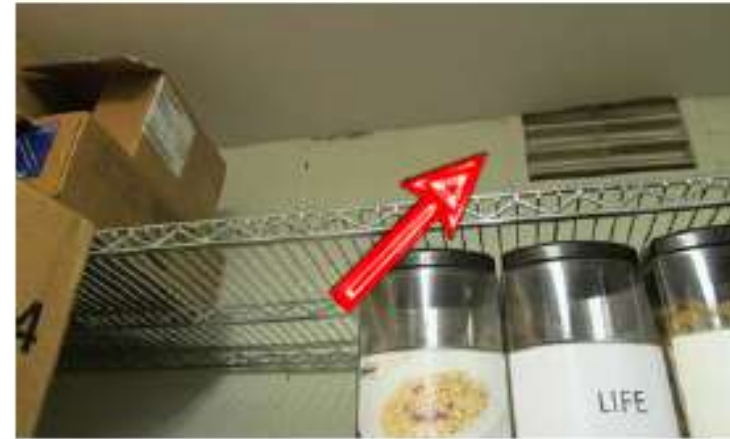
Image 2: Clean vents registers more often to reduce grease build up that can be a food sources to pests.
